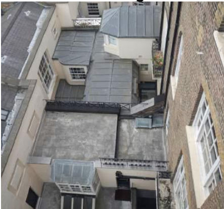
View of link building to rear of 144 Harley Street
